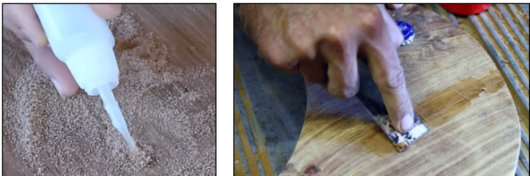
Figure 4: Using the Sawdust and Glue Mixture to Cover Wood Chipping.
