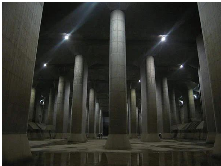
Fig. 2: The G-Cans project's water storage tank is supported by 59 pillars and stands at a height of 25.4 meters.
