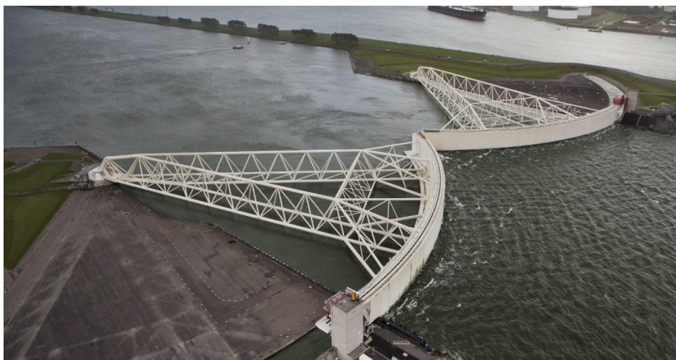
Fig. 3: The Maestlantkering is a storm surge barrier and a vital part of the Delta Works (Source: https://www.rijkswaterstaat.nl/en/projects/iconic-structures/maeslant-barrier )
