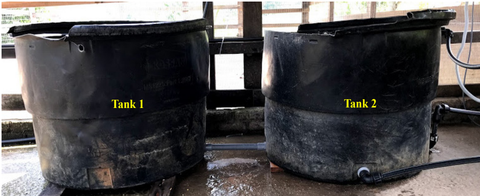
Figure 2. A two-tanks system was applied to ensure a continuous supply of water
