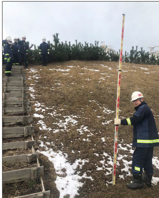
Figure 7. INPEX LNG regasification terminal - embankment between two plants
