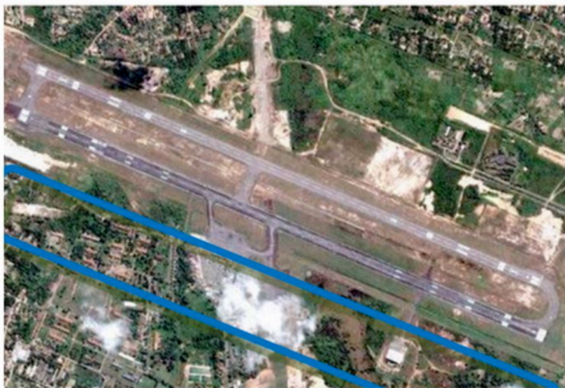
Figure 1. Aerial Photographs International Airport Sultan Mahmud Badaruddin II Palembang
