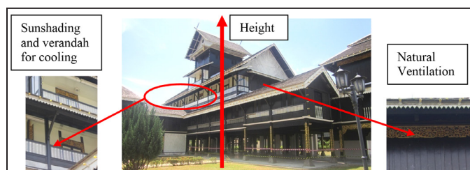
Figure 7. Images illustrating the passive design features of Istana Lama Seri Menanti
