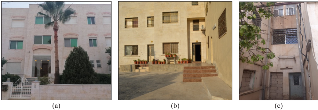
Figure 4. The main facades of the studied buildings: (a) Rectangular; (b) L-shape; and (c) U-shape
