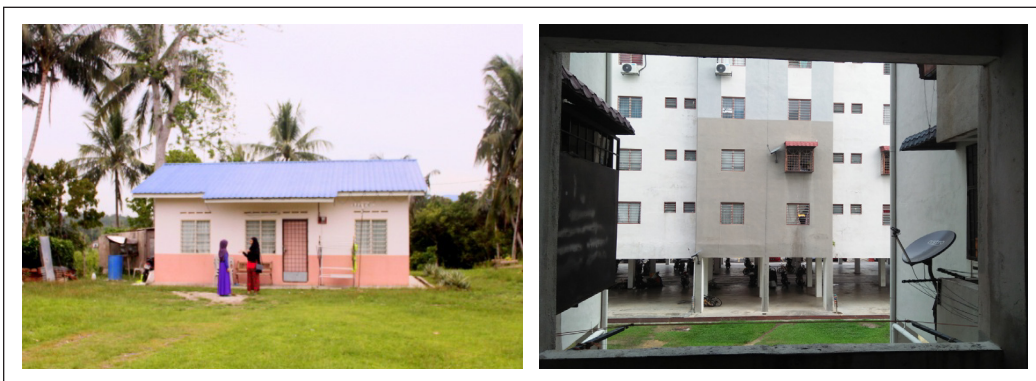
Figure 1. Single story, low-cost detached house with metal decking roof and plastered sand brick wall (Amir et al, 2019) (left), and high-density low-cost housing with air conditioning compressor on the facade (right)
