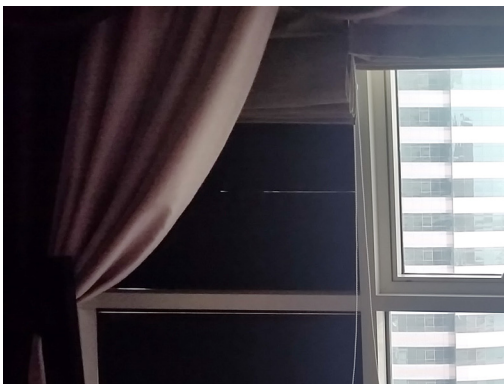
Figure 3. Window showing three layers of protection. 1. Insulation covering glass pane (the black surface behind the curtain and the blind) 2. Thick blinds, 3. Curtain (taken by the author, June 2016, Sharjah, UAE)
