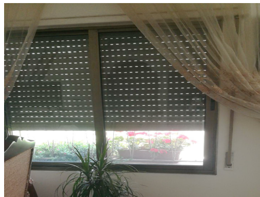
Figure 4. Exterior shutter from the inside. The strap on the right slides it up and down. The slits allow light in but close when the shutters are completely shut, thus improving insulation with the outside. (Taken by author June 2017, Amman, Jordan)
