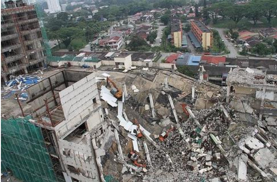
Figure 1.5 : Jaya shopping mall collapsing that happened in May 2009
