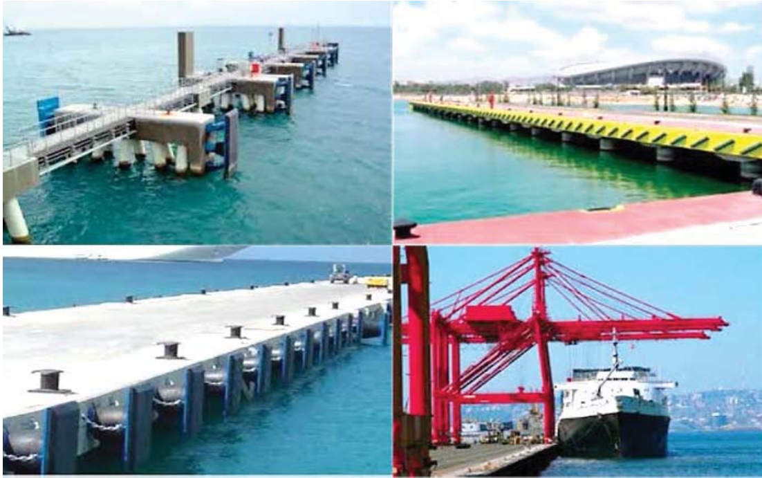
Figure 1.5 : Limited space at port and jetty.
