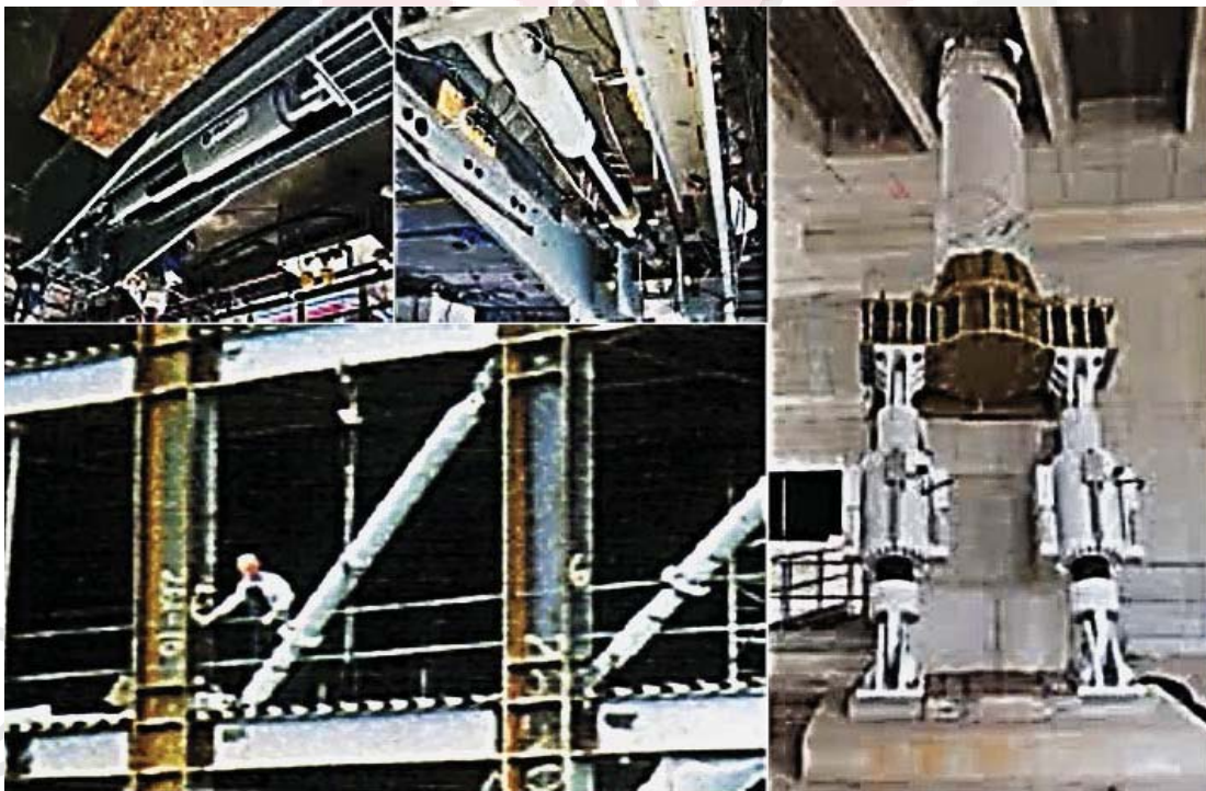
Figure 1.3 : Application of viscous damper
