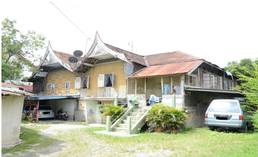
Figure 2. Renovated and extended (including building rooms with brick walls under the original on stilts traditional house) Traditional Malay House of Kelantan at Kota Bharu, Kelantan, Malaysia.
