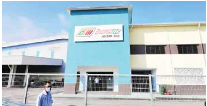
Diversatech Fertilizer manufacturing plant in West Port, Pulau Indah in Klang, Selangor
