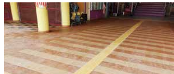
The disabled path in the Disabled (OKU) Student Complex which was completed in July 2023
