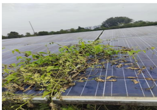
Fig. 7. Weeds growing on top of PV surface creating a permanent shading condition. The lining is used as quadrant reference for measurements.
