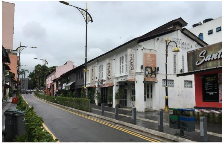
Figure 1.14 : Street and five-foot walkways at Jalan Dhoby
