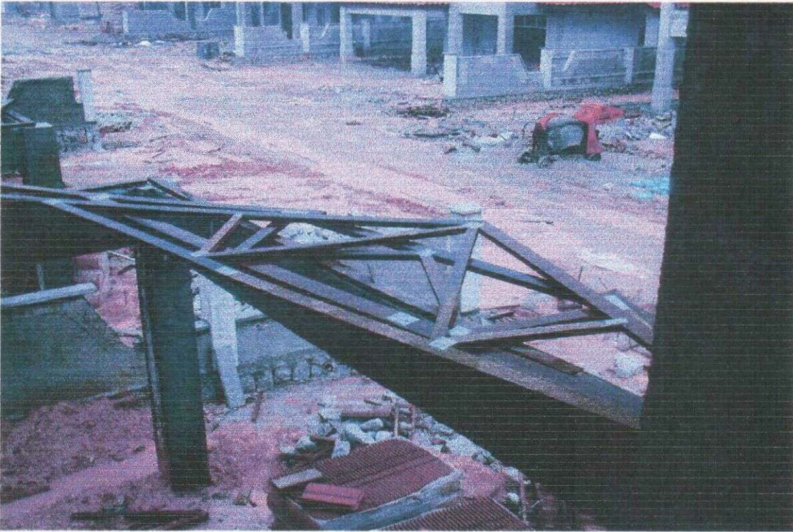
Plate 3 : Closer look at single unit of prefabricated timber roof truss framework
