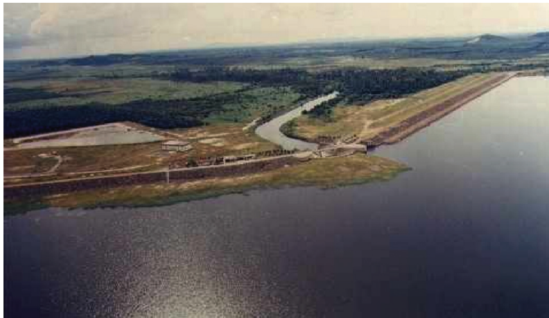
Plate 1: An aerial view of the Sembrong Dam and reservoir and the river downstream of the dam (Courtesy of Department of Irrigation and Drainage, Kuala Lumpur)
