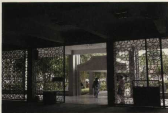
Fig. 5: Using passive ventilation for cooling buildings
