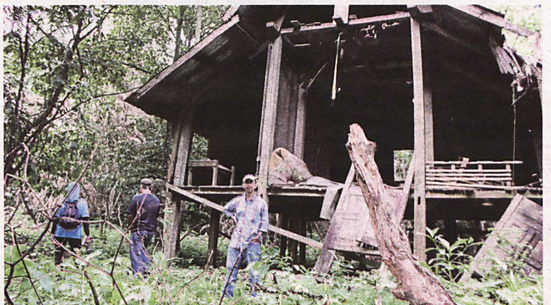
A house being dismantled for relocation.
