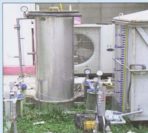
The treatment unit
