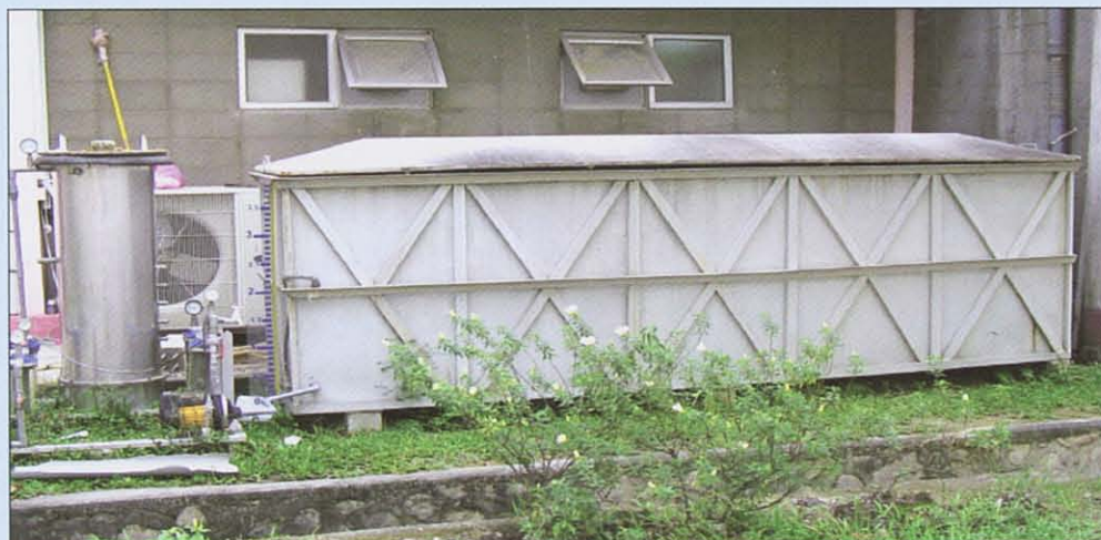
Rainwater harvesting tank and the treatment unit
