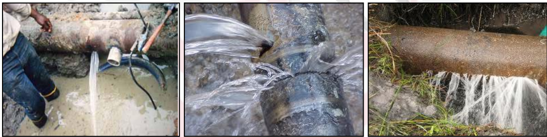
Figure 1.1 Examples of water leakage
