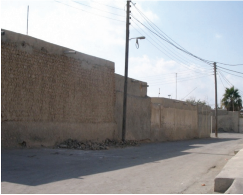
Fig. 16: A house without any outside opening, Old Saffein
