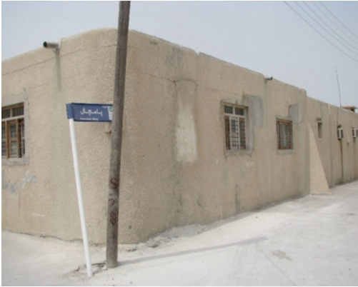
Fig. 17: Wider openings built at New Saffein
