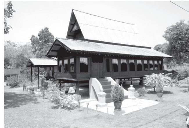
Figure 1: A renovated house sponsored by PERZIM (Source: Author)
