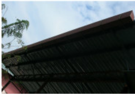
Figure 4: Picture of 140 mm x 140 mm gutter.
