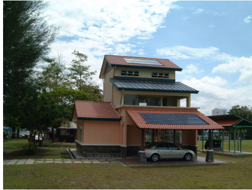
Figure 5: Building Integrated Photovoltaic. (Source: Solar House, SIRIM Bhd., Shah Alam)
