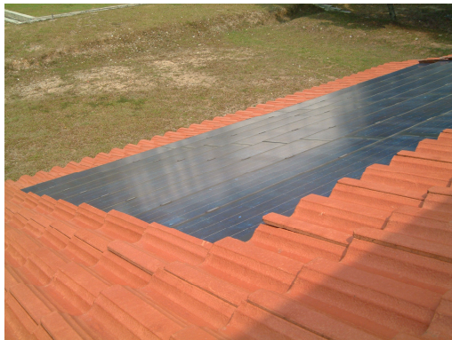
Figure 6: Building Integrated Photovoltaic for Roof Tiles (Source: Solar House, SIRIM Bhd., Shah Alam).
