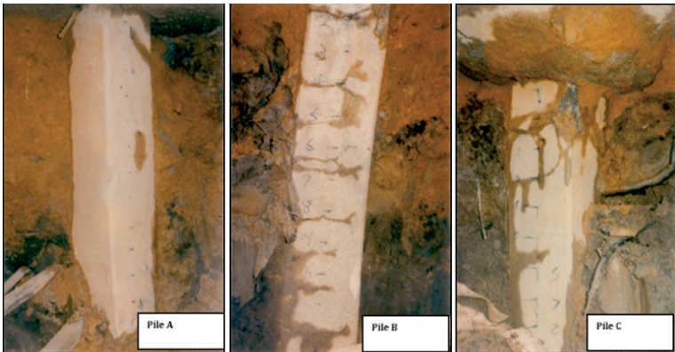
(c) Bridge pile failures, attributed to soil lateral movement (Gue & Tan, 2003)
