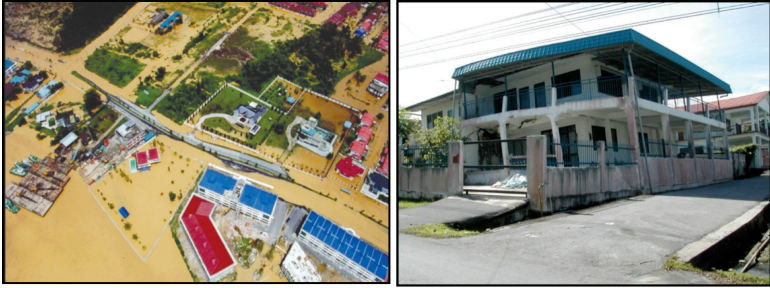
(b) Flooding and damage to infrastructure in Sibu Town (Sarawak), both attributed to subsidence of peat upon which most of the town was built
