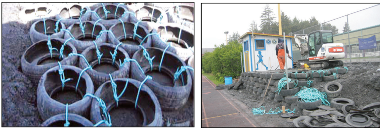
(a) (b) Figure 59 Scrap tires retaining wall: (a) tires with one side wall removed tied with polypropylene ropes, and (b) wall construction in progress
