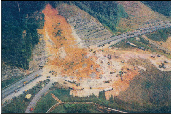
(c) Deep seated rotational slide of an 'engineered' anchored slope at Gua Tempurung, Kampar, Perak in January 1996. 1 person died
