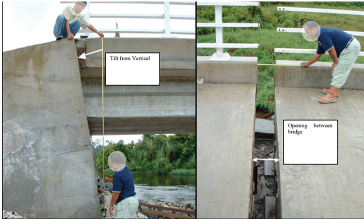
(d) Abutment tilt and gap between bridge decks due to foundation failure on soft ground (Gue & Tan, 2003)
