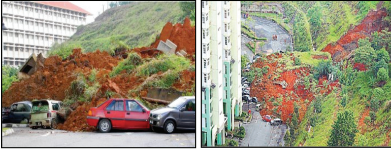
(g) Landslide on March 22, 2007, Precinct 9 Putra Jaya after a period of heavy rain. 23 cars were buried under the rubble. 1200 people were evacuated (Photos courtesy of the New Strait Times)
