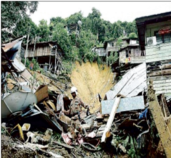
(h) Landslide at Kampung Cina, Kapit on December 27, 2007 during a heavy downpour. 12 houses were destroyed involving 17 families (76 people). 9 were injured, 4 were lost
