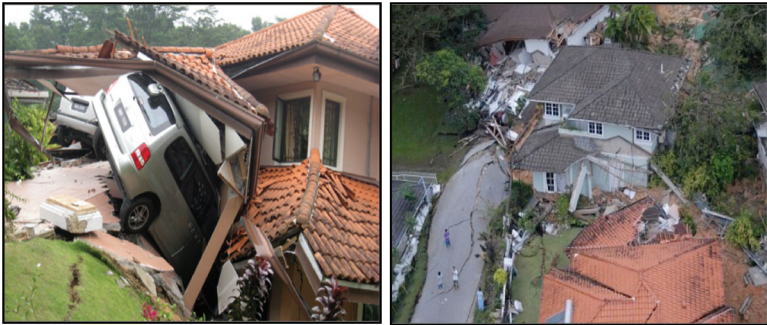
(j) Landslide at Bukit Antarabangsa, Kuala Lumpur (an up-scale residential area) on December 6, 2008. 5 people died (photo courtesy of Google)
