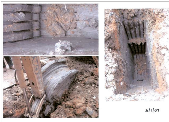
Figure 11 Soft marine clay revealed during excavation work carried out in January 2007
