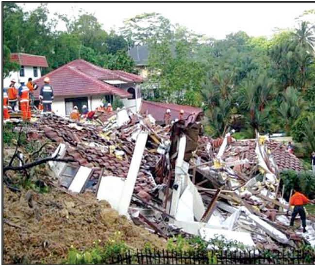
(d) A bungalow house at Taman Hill view, Ulu Klang, Kuala Lumpur dilapidated by landslide in November 2002. 8 people were killed
