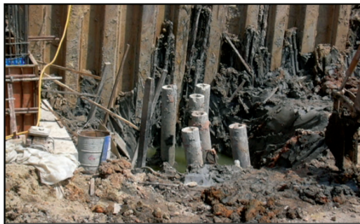
Figure 8 Pile failure in an open excavation
