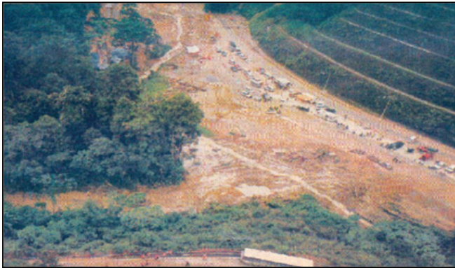
(b) Debris flow during heavy down-pour at the Karak Highway – Genting Highland slip road (road to one of Malaysia’s top hill resort destinations) in June 1995 killed 22 whilst 23 others were injured
