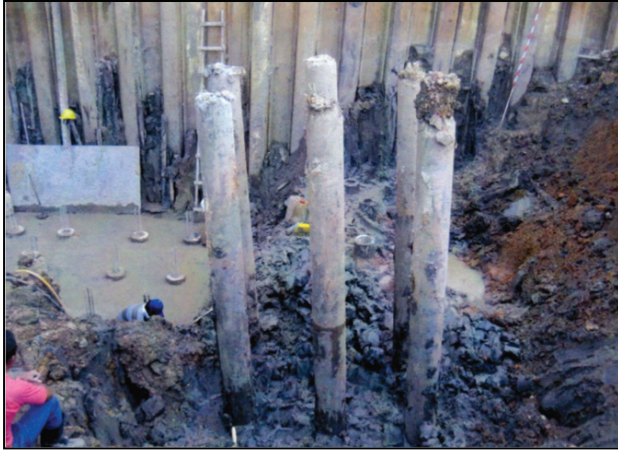
Figure 13 Broken piles P1, P2, P3, P5 and P6
