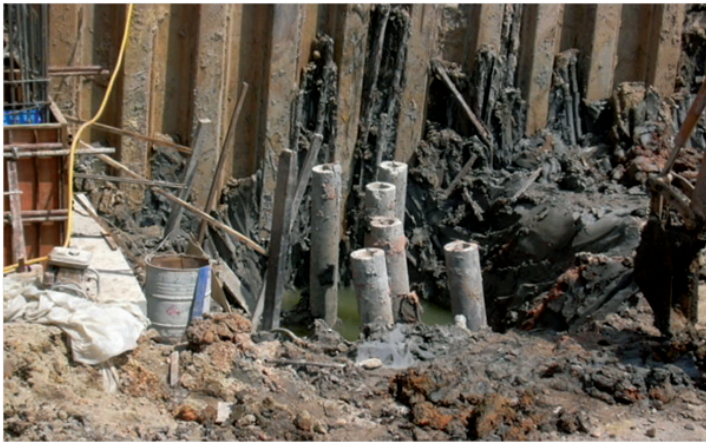
(e) Pile broken due to excessive lateral movement of soft soil in open excavation during construction of a lift shaft for the Majestic Hotel, Malacca, 2007
