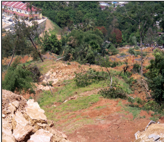
(f) Landslide at Kampung Pasir, Ulu Klang, Kuala Lumpur in May 2006. 4 were killed when one longhouse was buried under the avalanche of earth debris
