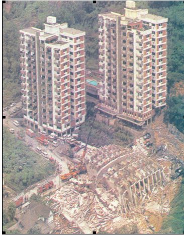
(a) Collapse of the Highland Tower, Ulu Kelang, Selangor in December 1993. 49 lives were lost, only 2 survived, a maid and a baby girl. Fortunately most of the occupants were at-work at the time of the disaster. The remaining 2 blocks have been left unoccupied till today
