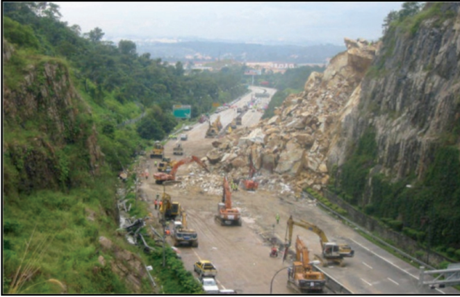
(e) Rock fall at Bukit Lanjan, New Klang Valley Expressway, Selangor in November 2003. A major rock fall in the country which led to closure of one of the main gateways to Kuala Lumpur for more than 2 months
